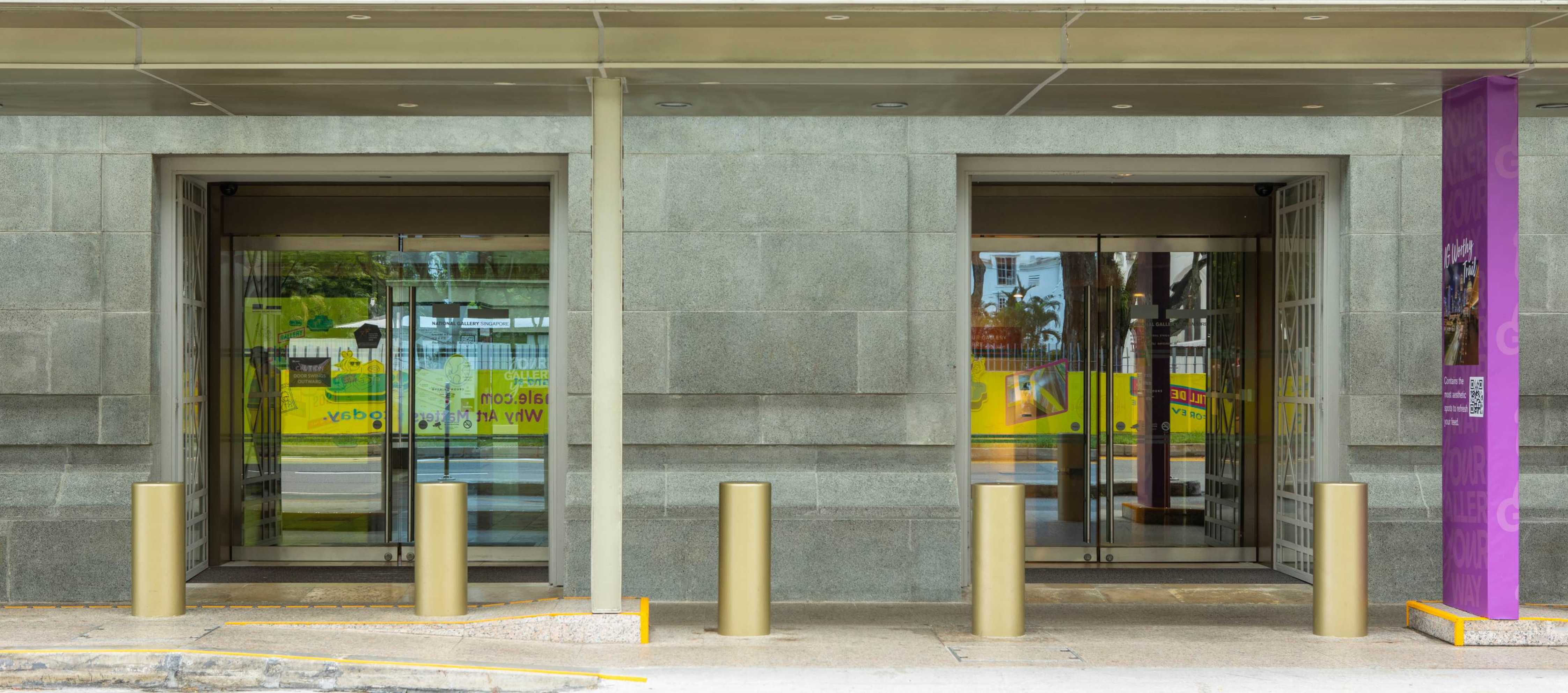
Doors closed at Coleman Entrance
