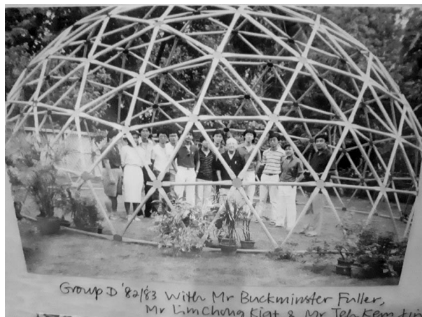
Pipe geodesic dome at Starpoint, 1982.
