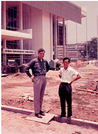
Engineers Povl Ahm and Hou Ke-Hua in front of the Singapore Conference Hall
