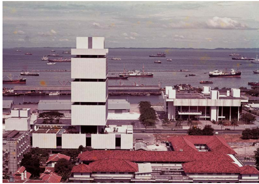
The now demolished MSA building (left) and Singapore Conference Hall (right)
